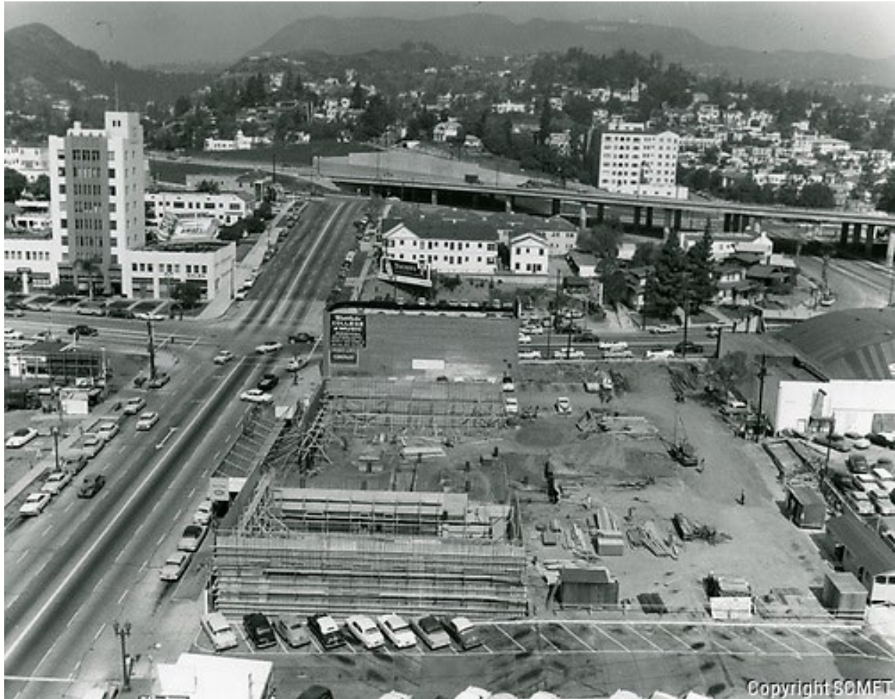
Figure 2: Base of Capitol Tower under construction, view looking north, 1955. (SCMFT)
