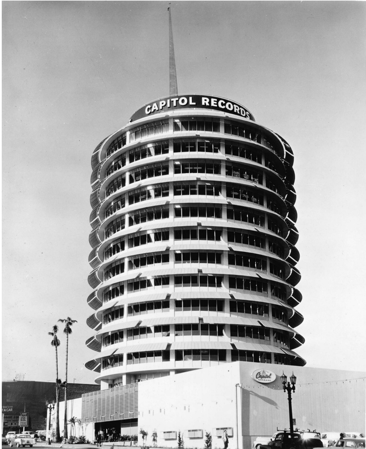
Figure 6: Completed Capitol Tower, 1956. (USC: California Historical Society Collection)
